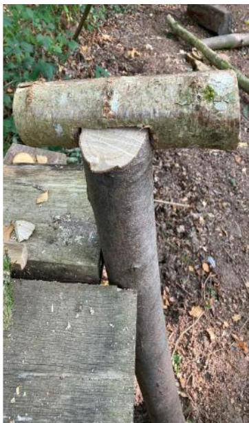
sample pole and ridge joints- sweet chestnut and hazel.
