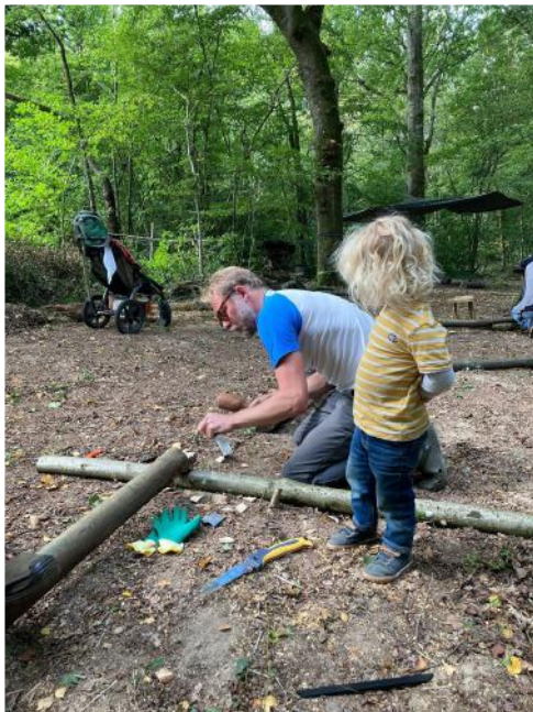
chiselling ridge pole joints
