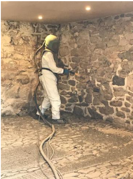
3 rd April 2021: the Grade II listed cobbled dairy had to be retained as a historically integral part of the building. However it was sandblasted, enabling the room to be converted into a useable sitting room with a gently sloping floor.
