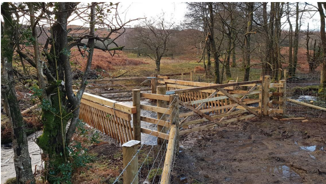
Figure 3: Newly installed crossing point for livestock and vehicles.
