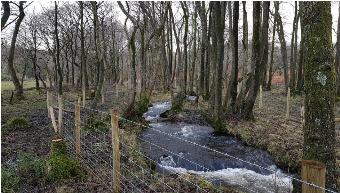
Figure 2: Newly installed fence line to reduce livestock poaching, sedimentation and nutrient inputs to Spannel Beck.
